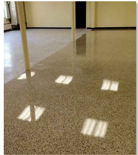
Terazzo Flooring Coated With X-PROTECT TILE & GROUT - High Gloss (Before & After Comparison)
